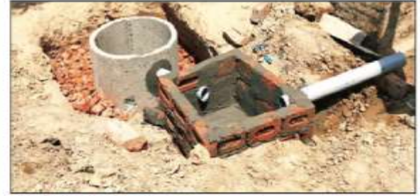
A soak pit in one of the houses of Man Aspal village
